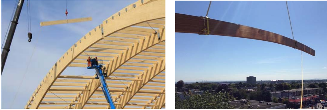
Figure 5.3 Lifting Lam+ beams with a crane
