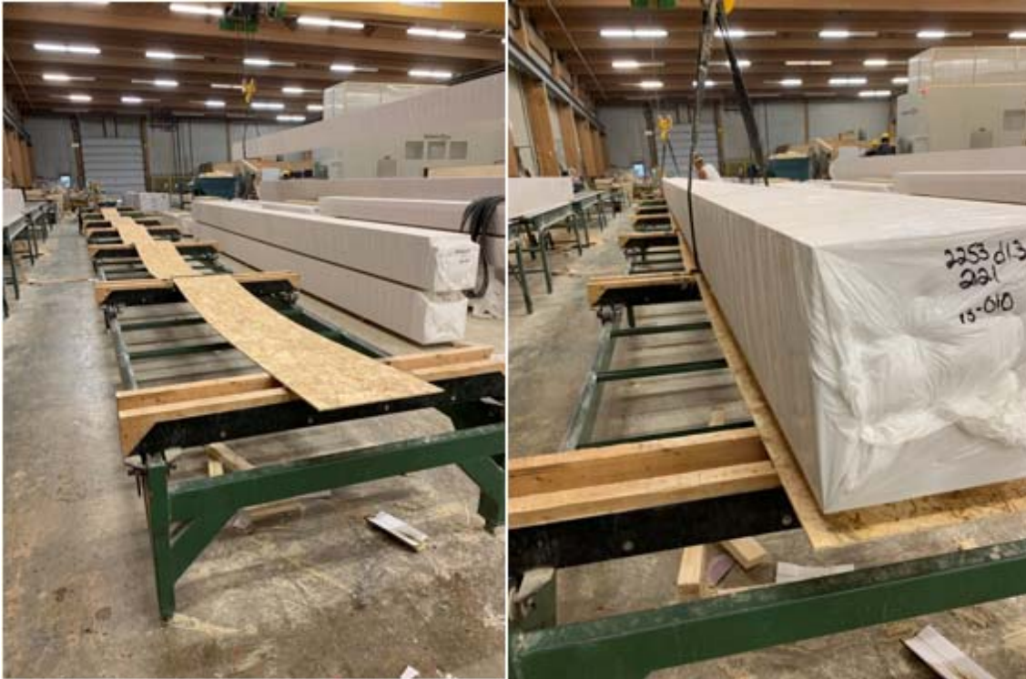
Figure 4.14 OSB is then placed on equally spaced lumber supports and the wrapped glulam members are stacked on top. For greater stability and safety during handling, glulam members are stacked lying flat.
