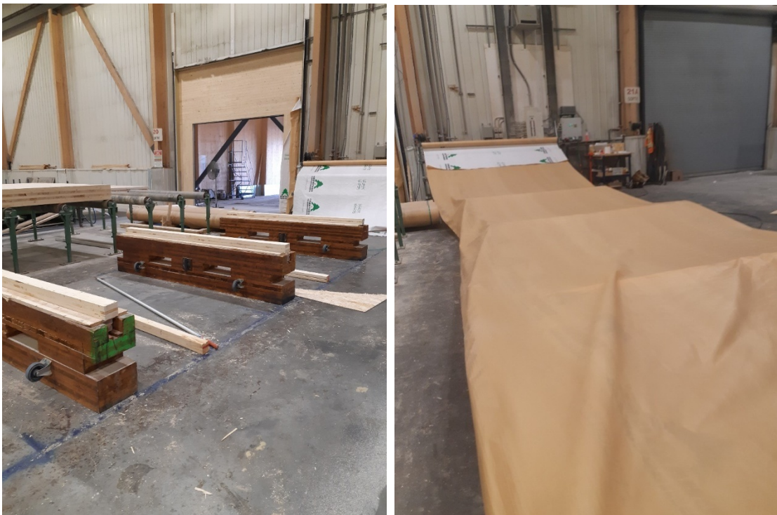
Figure 4.3 First, wrapping is unrolled over lumber blocking which has been placed on lumber supports.
