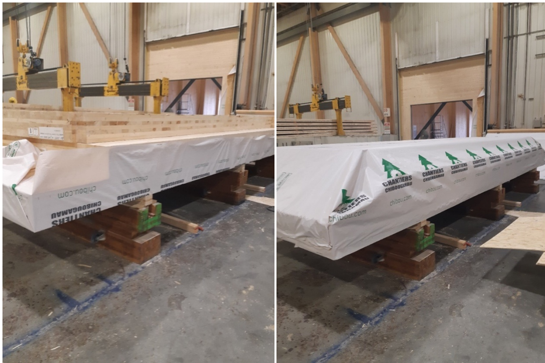
Figure 4.5 The protective packaging is then wrapped over the panels and stapled.
