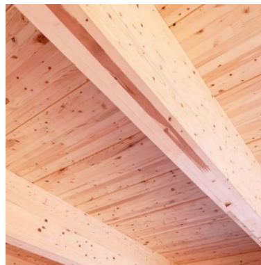
Figure 3.11 Coloration du pin gris
