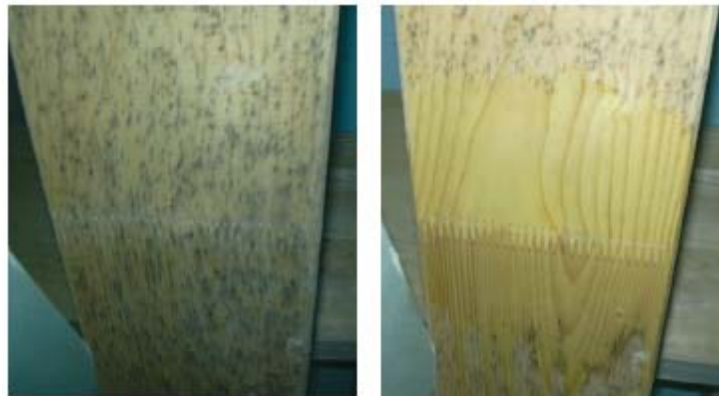
Figure 6.3 Iron stains (left) and treatment with oxalic acid (right)
