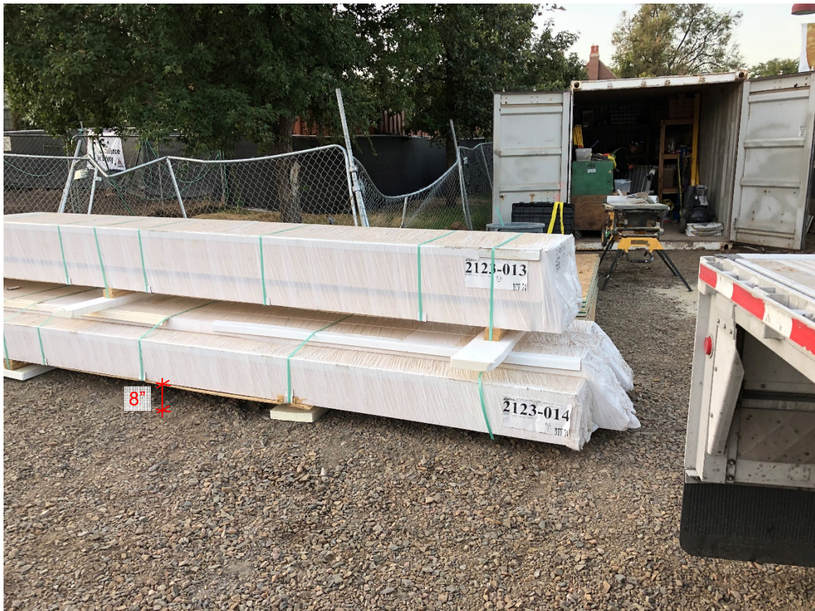
Figure 4.18 Proper storage of products on lumber blocking to ensure good airflow
