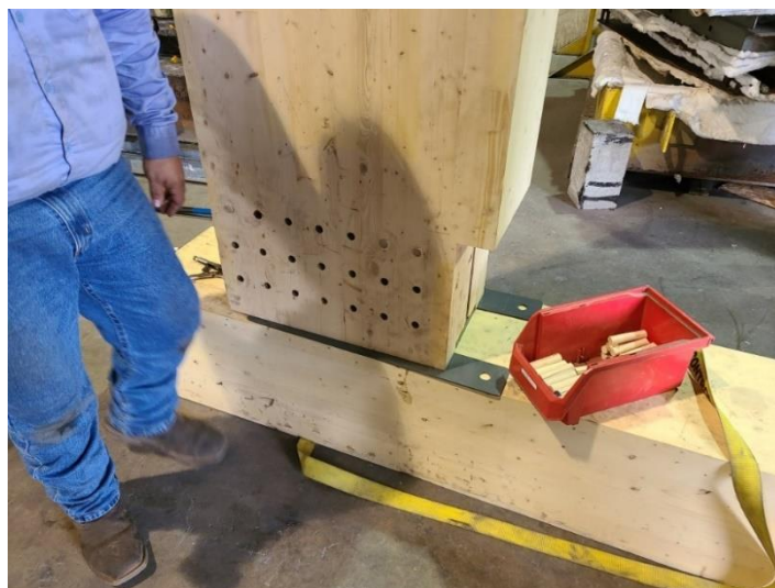
Figure 2: Beam (vertical) and column (horizontal on floor) during installation of wood plugs.
