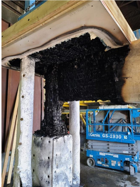
Figure 12: Test assembly post-test
