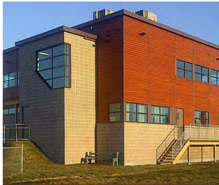
Recreation centre Saint-Prime, Que. (2011)
