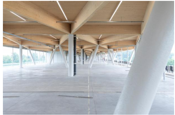
Figure 5 – Steel Structure with Intumescent Fire-protective Coating
