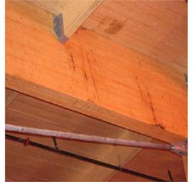
c) Rust marks caused by the use of a grinder to cut steel near a wood column: particles of steel get lodged in the wood, and begin to show when oxidation sets in a few weeks later
