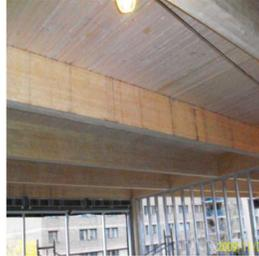
d) Mold due to a long period of storage on the building site without proper ventilation (Nordic systematically ventilates the timber it delivers using wood spacers intended for this purpose)
