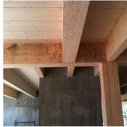
e) Marks from straps used during lifting or wood spacers placed on the ground
