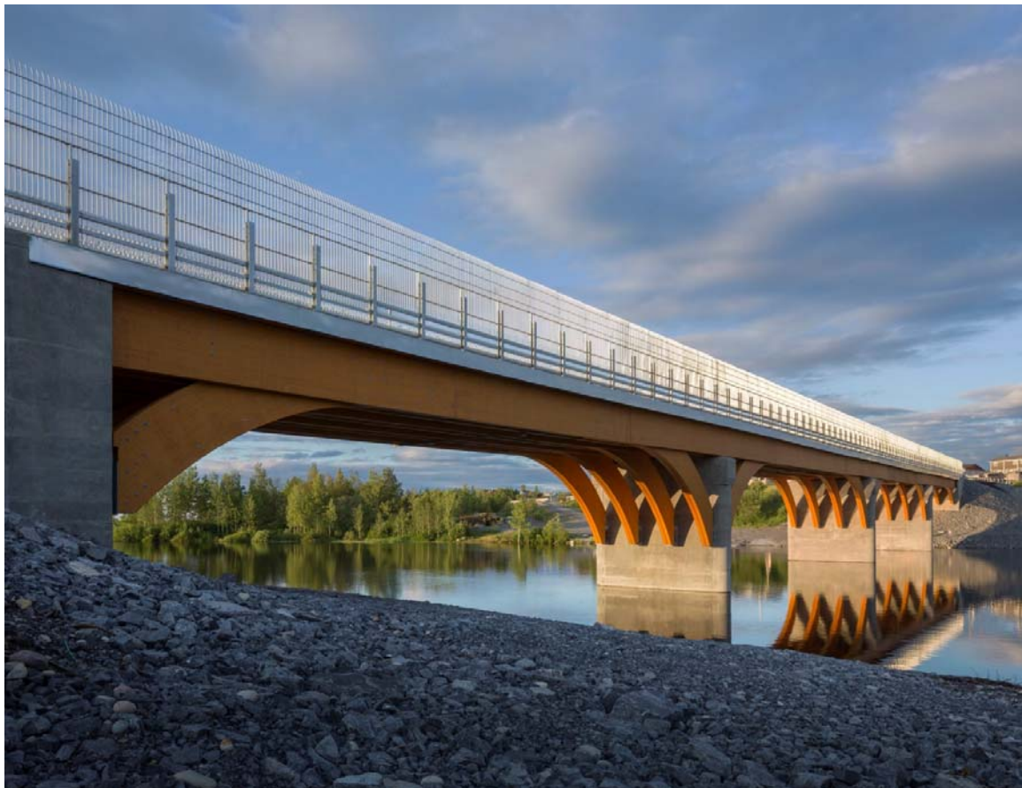
Figure 16: View of the bridge from east bank
