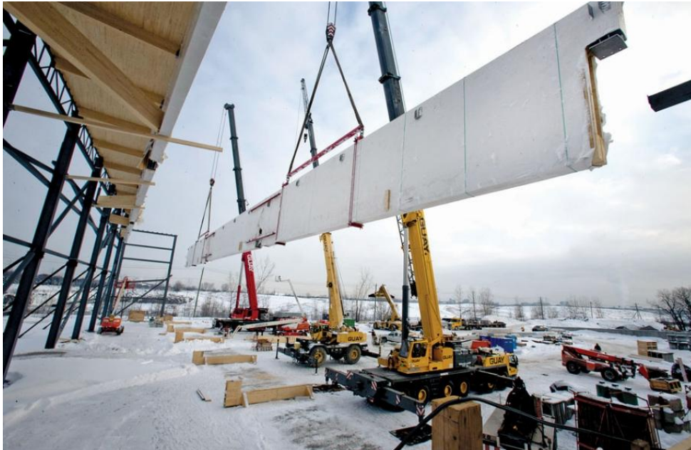
Figure 21: Installation of the second principle beam
