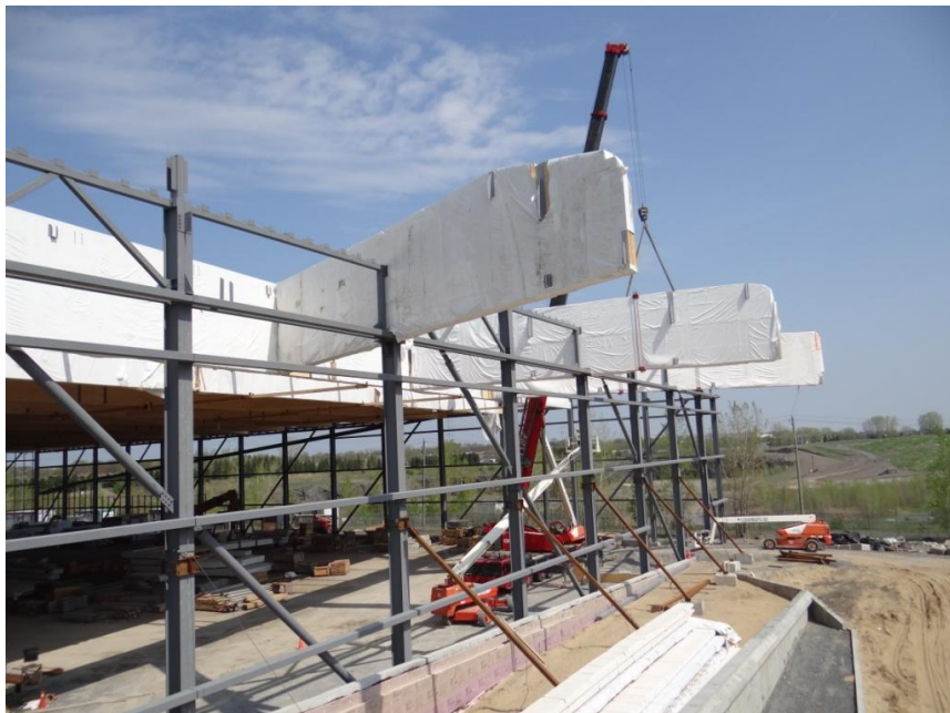
Figure 22: Installation of the cantilever beams
